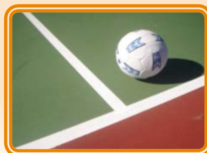
Well installed line marking – crisp & sharp edges
