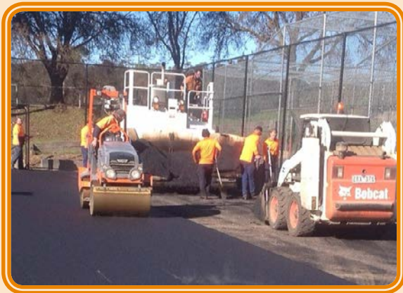
Asphalt paving machine
