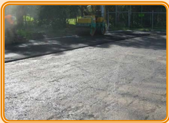
Prime coat on the FCR
