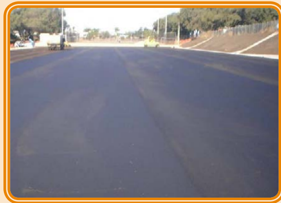
Asphalt laid in runs
