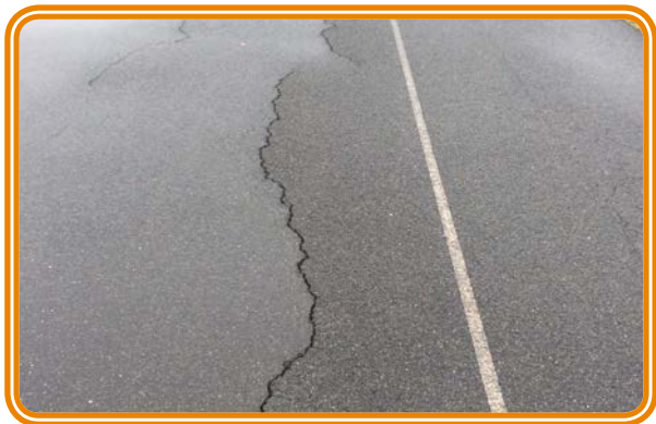
Asphalt cracking
