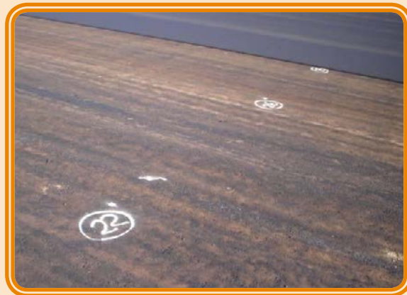
Surveyed and marked
