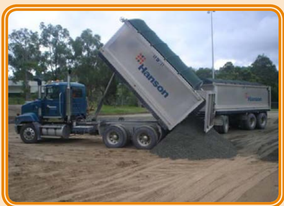
Importing the crushed rock layers – sub-base
