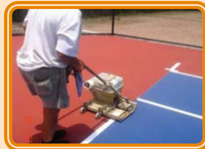
The gravity fed line marking machine method
